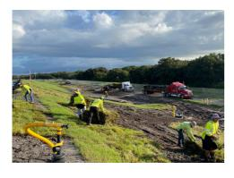
Local landfills use sod as a means of erosion control on a regular basis. The EPA regulates the maintenance of a municipal solid waste landfill to prevent pollution. As such, there are areas that are constantly being reworked, or newly filled areas that have reached its maximum capacity that must be capped and sodded in order to comply with regulations.
